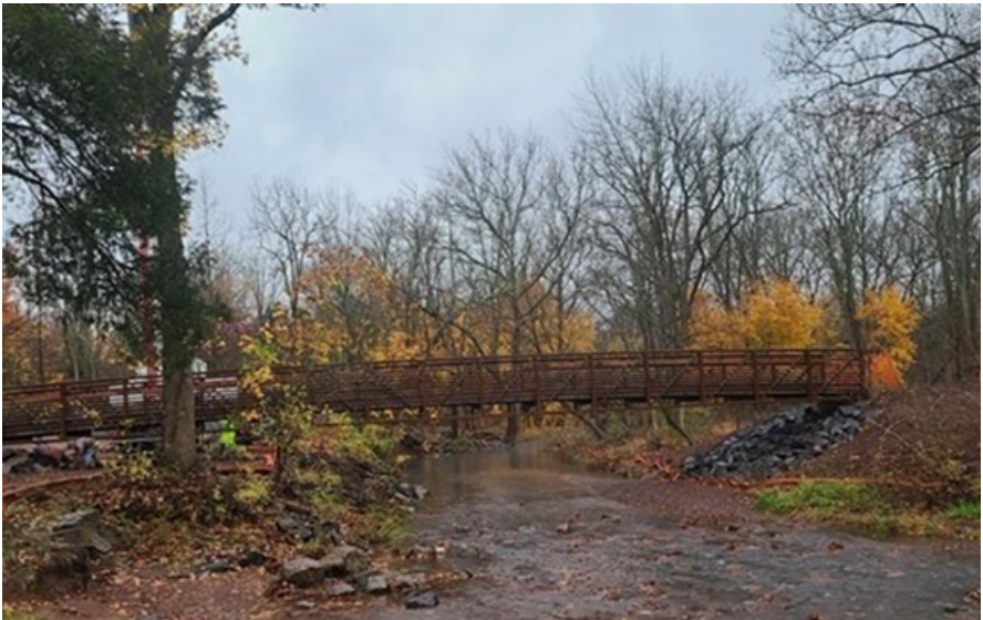
Example of a pedestrian bridge to be built next to the foundations of the old bridge
