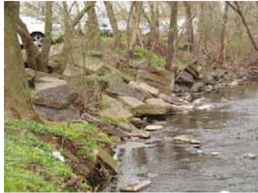
Figure 6 - Concrete Debris along banks of Creek in Newtown Borough
